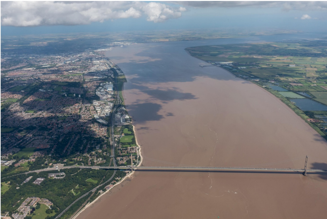
Hull and the bridge
