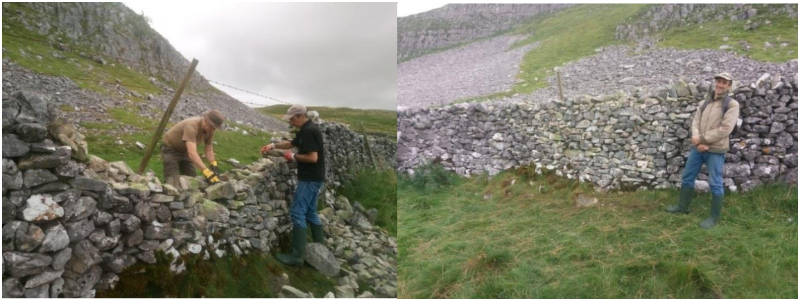
Wall repair , Photos: Ed Cleasby
